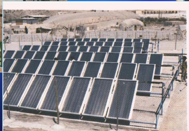
MOSALA(MOSQUE) OF ZABOL SOLAR HOT WATER SUPPLY
